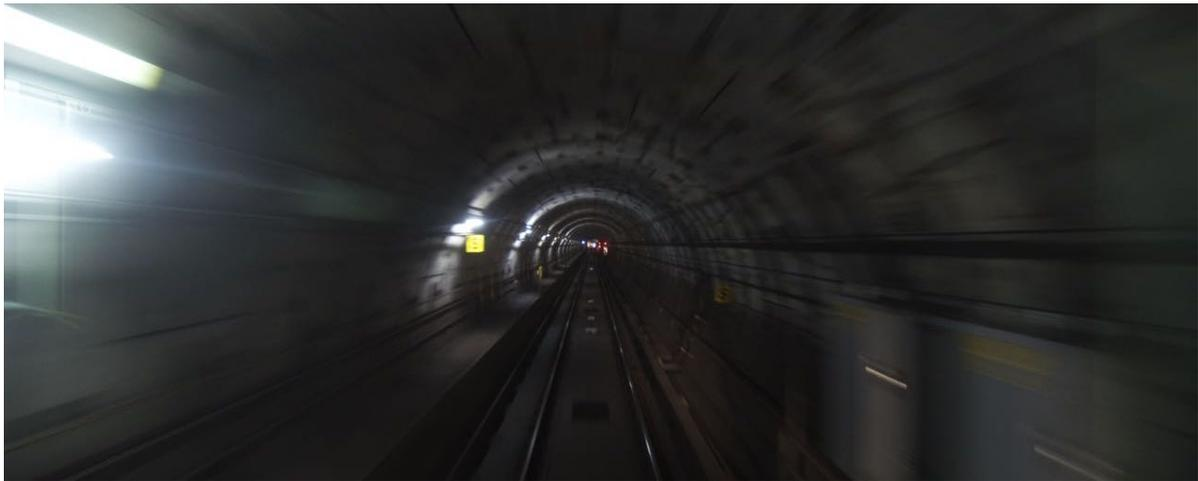
Figure 1.2: Picture of an underground tunnel connecting two subway stations. It highlights some of the pathological conditions for localization that need to be addressed (e.g., low light, smooth wall surfaces and motion blur).
